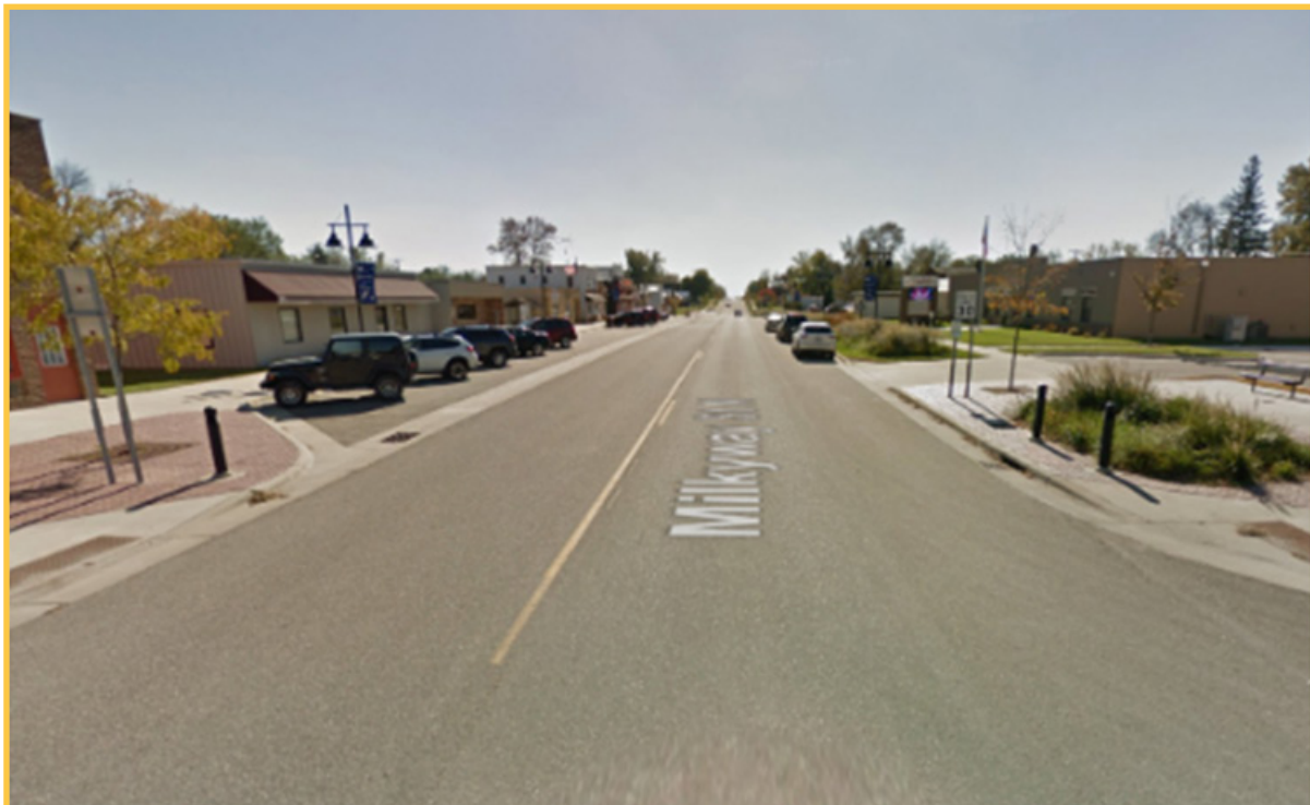
Curb Extension in Cosmos, MN
