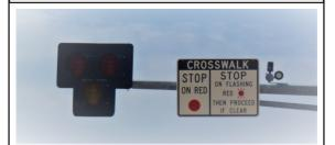
A **HAWK** (High-Intensity **A**ctivated cross**W**al**K**) signal is a signal-beacon designed to help pedestrians safely cross busy streets.
