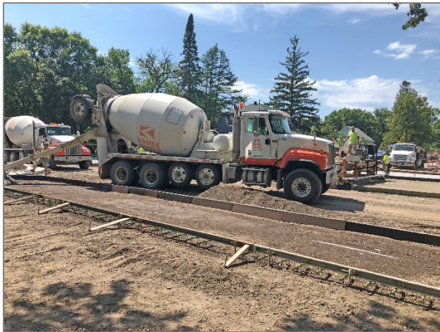
Photos above: (left) cement trucks delivering concrete to the roadway; (right) new concrete pavement on Highway 15 between 4 th Avenue South and 5 th Avenue South.
