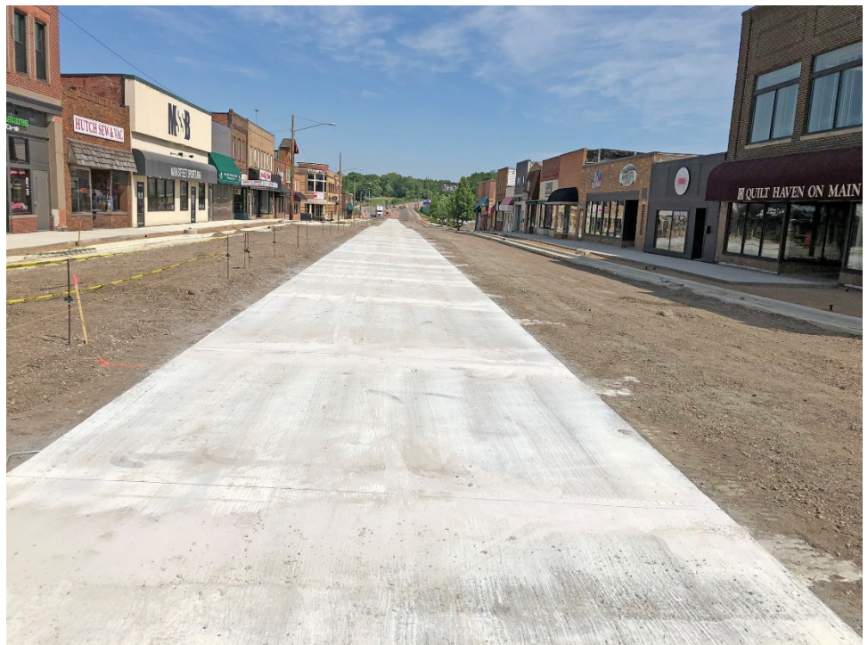
Photo above: the completed 13-foot concrete middle lane.
