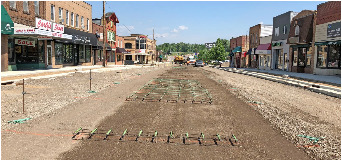
Photo above: Preparing for the middle lane concrete pour.
