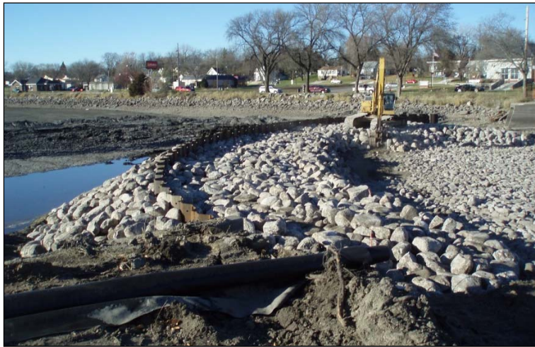
Figure 1 - Steel Sheet Pile Weir
