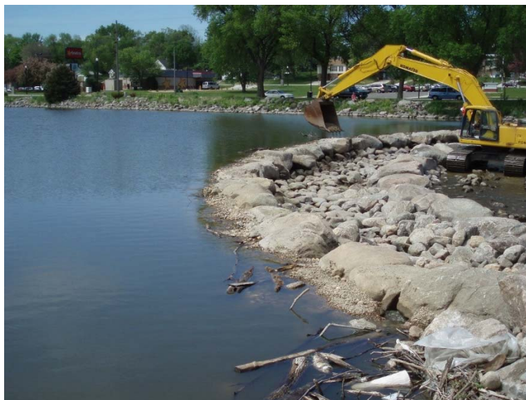
Figure 3 - Placement of Chinking Rock
