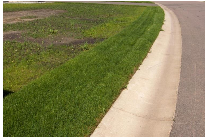
Established grass buffer strip. These should be left undisturbed until the final lot grading and sodding or seeding.
